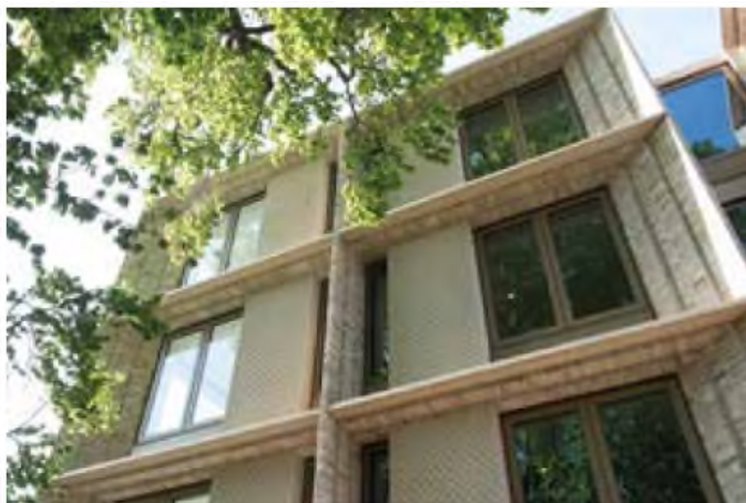
Exterior of Block A at the Master's Field, the first of ten blocks to be completed as part of the development. Photograph by Rob Judges.
